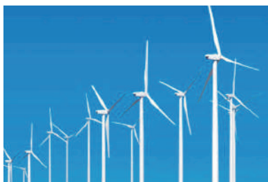
Wind Power Generation
